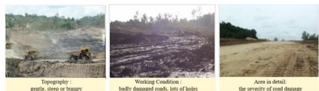
Fig. 7. Photo documentation of working condition
