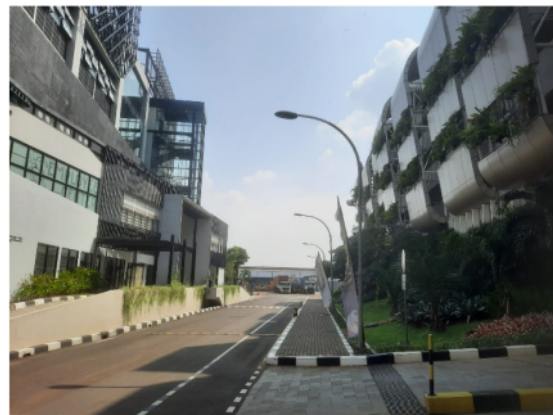
Figure 12: Tunneling Effect Between Two Large Buildings Resulting Higher Wind Speed Measurements.
