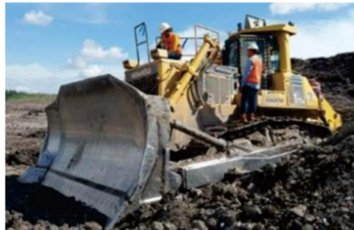
Fig. 1. Several technicians are handling a bulldozer that was damaged while operating in the field.
