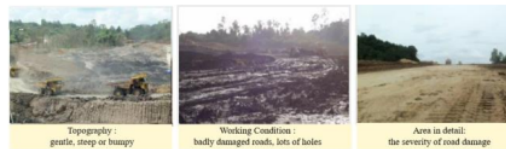
Fig. 7. Photo documentation of working condition
