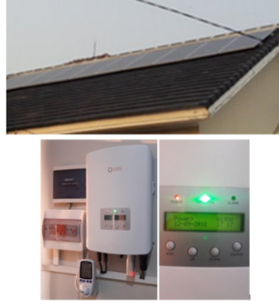
Fig 3. Installation of a rooftop solar panel PV system on site for the test.
